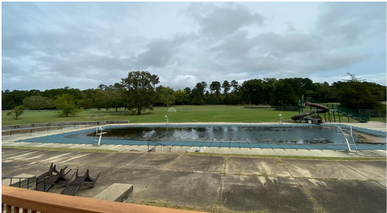
Figure 7: Defunct pool identified from a third-party inspection; repairs not planned due to high restoration costs
