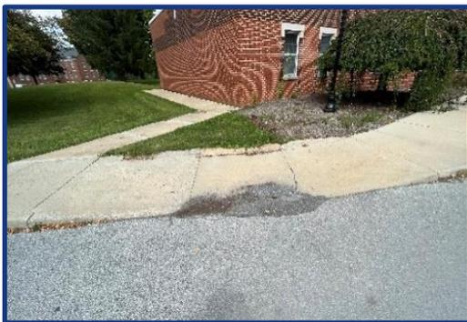
Figure 2.1: Uneven surface and steep slope
