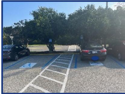
Figure 3.1: Low parking signs and inadequate access aisle width and location
