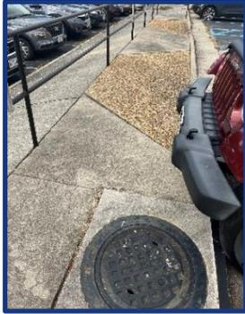
Figure 2.3: Parking lot contains uneven surfaces and changing slopes
