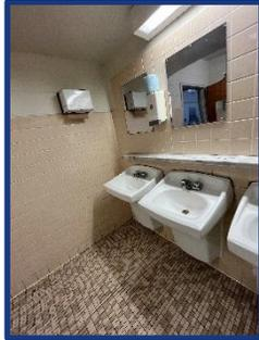
Figure 9.1: Mirror improperly positioned, hand soap and towel dispensers exceeding reach range
