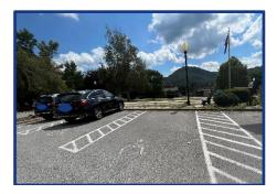
Figure 3.3: No parking signs, no van accessible spaces, and inadequate access aisle width
