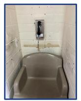
Figure 4: Floor space under telephone obstructed
