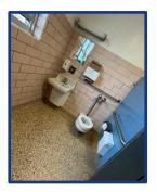
Figure 9.2: Mirror improperly positioned and hand soap, towel dispensers, and grab bar exceeding reach range
