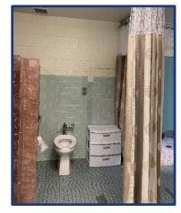
Figure 5: Toilet compartment wall replaced with a floor to ceiling curtain
