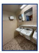
Figure 9.1: Mirror improperly positioned, hand soap and towel dispensers exceeding reach range
