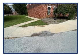
Figure 2.1: Uneven surface and steep slope
